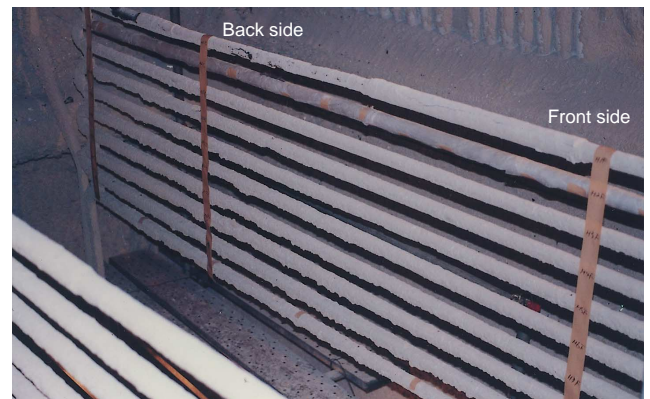
Fig. 5. Appearance of the counter-flow type superheater for 450 steam at the incinerator run down. ( May '97 )
